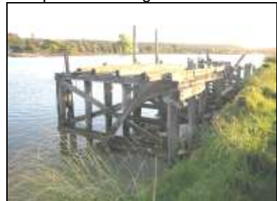
Old Gas Works Wharf
