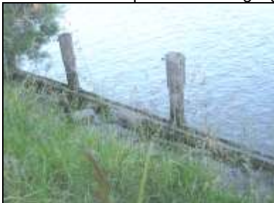
Old wooden breast work foundation
